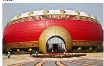
■ Largest drum-shaped building in Hefei sets Guinness record
